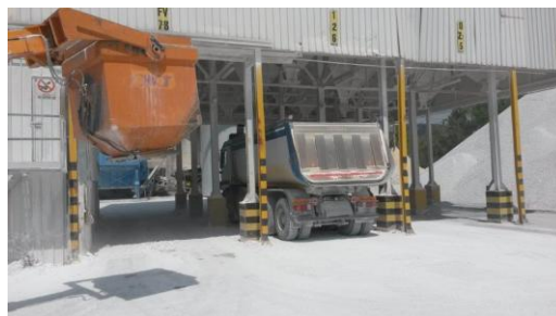
Storage in silos of fine material
